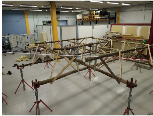
Figure 9: First steps of construction
