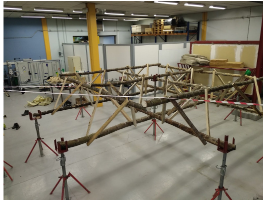
Figure 9: First steps of construction
