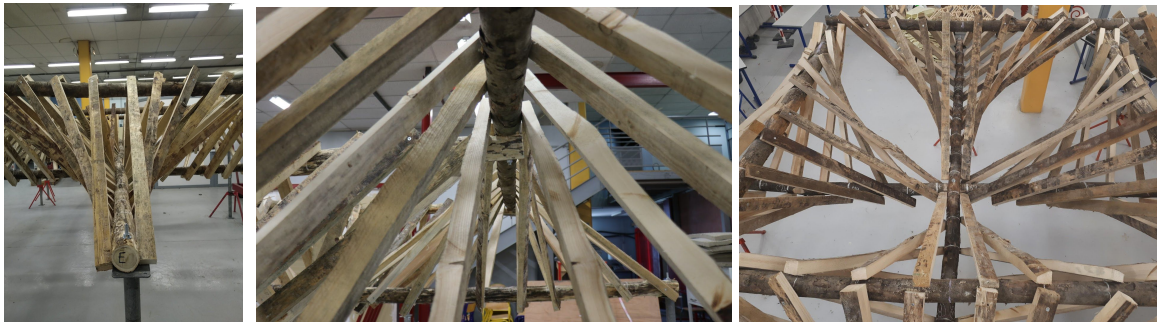
Figure 10: Different views of the constructed truss
