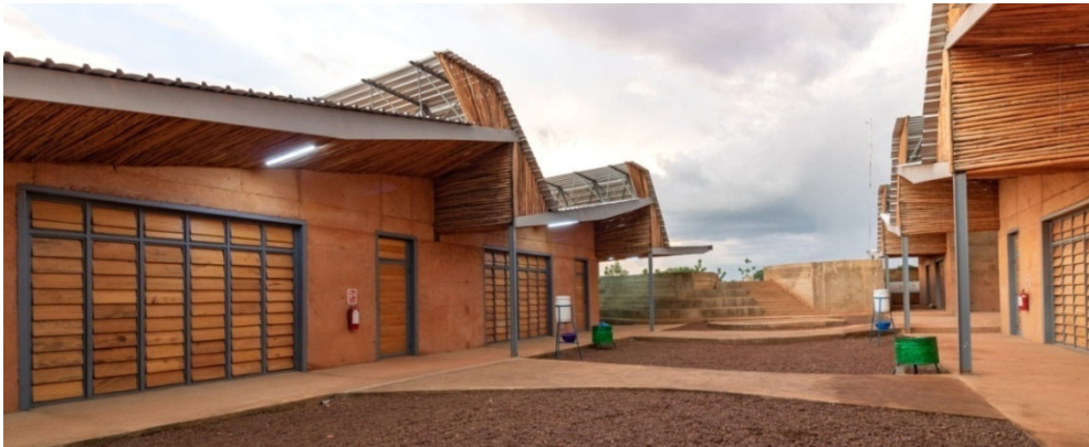
Figure 13 Burkina Institute of Technology (2021), Koudougou, Kere Architecture - Keré Architecture
