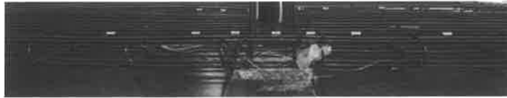
Figure 4. View of the fiber sensing rebars, installed within the mock-up prior to pouring of concrete (FBGs are identified by white markers).
