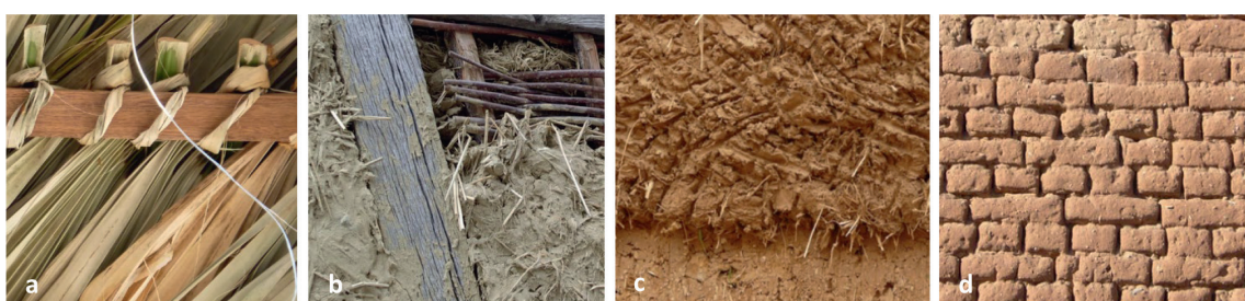
Figure 3. Raw plant fibers in building materials: a-roofing, b-cob and wood, c-cob wall and d-adobe bricks.
