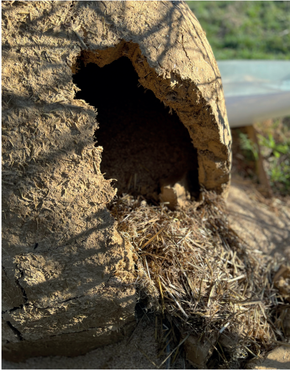
Figure 10. January 2022, the second silo prototype ripped open. © Aurélie Feuillas.
