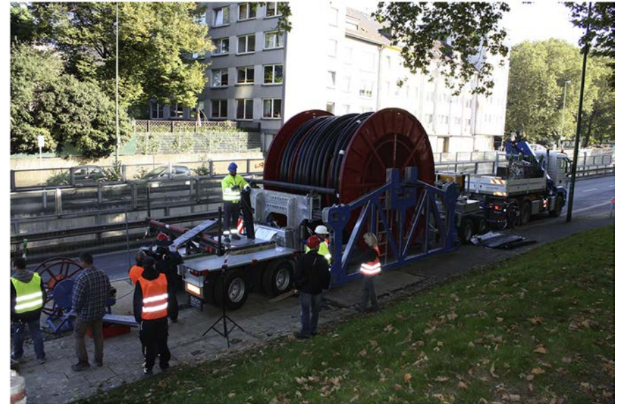
Laying of the AC HTS cable into its flexible cryostat for the Ampacity project.
