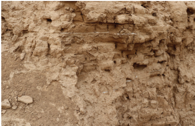
Figure 10: Borsippa: reed mats in earth masonry. © A. Al Taei
