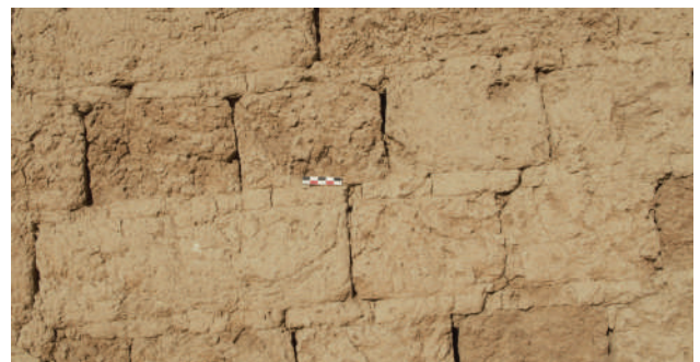
Figure 6: Detail of the facing: the horizontal joints have an even thickness of about 2 cm, while the vertical ones are much thinner.
