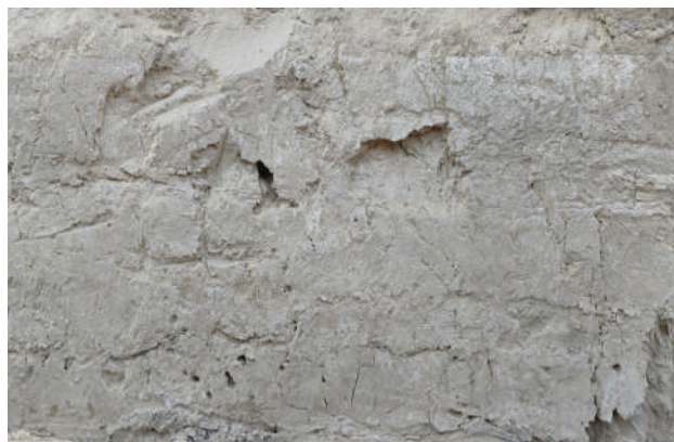
Figure 3: Babylon Ninmakh temple. Lime plaster. © A. Al Taei
