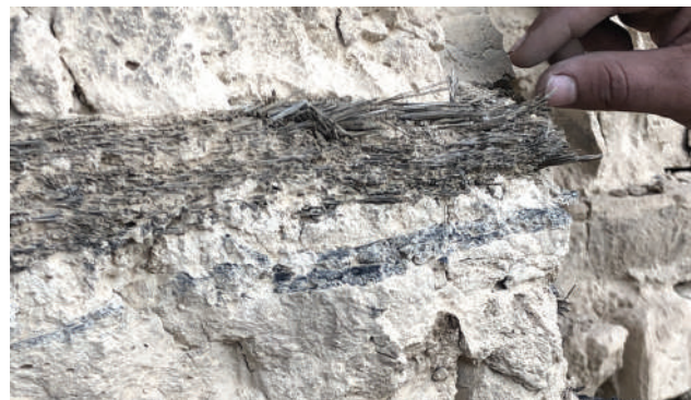
Figure 8: Borsippa: reed mats and bitumen layers in brick masonry. © A. Al Taei
