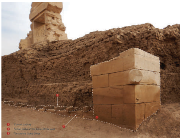
Figure 10: Stone reinforcements in the wall. © M. Vanpeene
