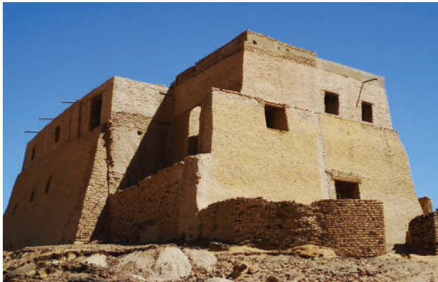
Figure 1: View of the mosque in Old Dongola. © K. Wasilewski
