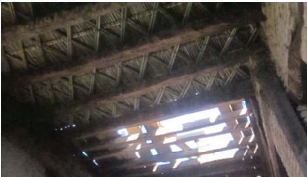
Figures 11, 12, 13: Show the different roofing processes. © M. Mohamed
