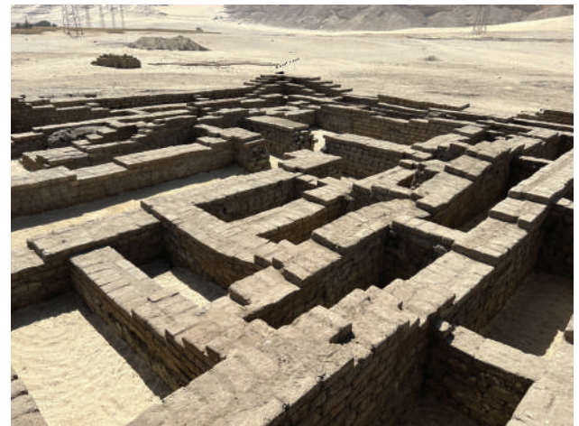
Figure 6: Existing walls, stabilized walls, and restored walls in the north section of the Pyramid.
