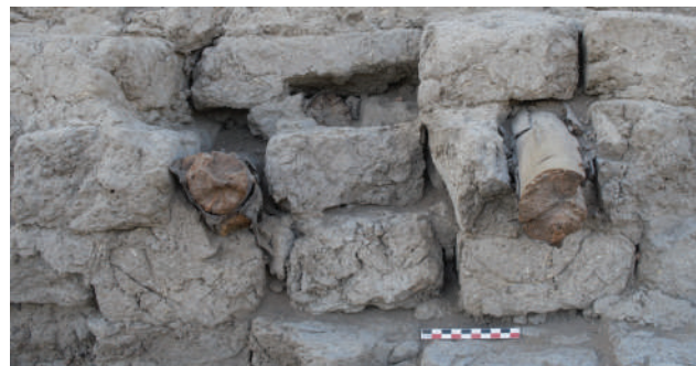
Figure 9: Wood reinforcement in the masonry. © M. Vanpeene
