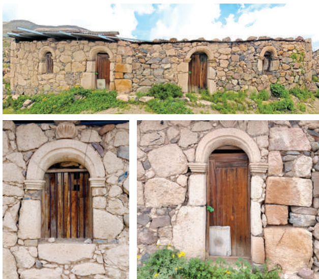
Figure 12: Housing Typology 3. Stones set in clay mortar and details of arches, imposts and ornaments carved in limestone. © J. Quiroz Bravo, 2019
