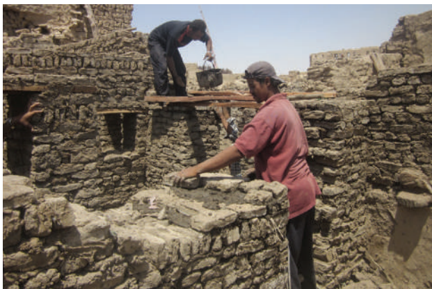
Figure 9: Wall construction process. © M. Mohamed
