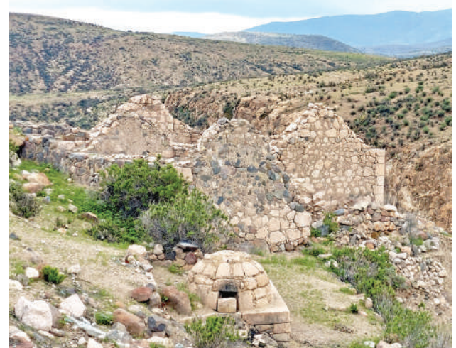
Figure 6: Houses and oven made of earth and stones. Village of Sipiza. © J. Quiroz Bravo, 2023
