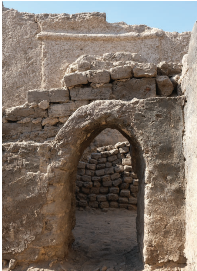
Figure 13: Gallery 24, doorway 24, from East.
