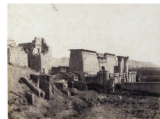
Figure 6b: F. Teynard (calotype pl. 34): Medinet Habu, East gate leading to Migdol, looking to S-E. © N. Lienhard (CRES)
