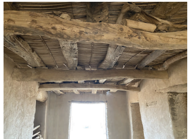
Figure 8: Reuse of a wooden boat as a roofing material. © PCMA, UW, T. Fushiya
