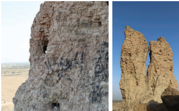
Figure 11: Ventilation channels in brick masonry. © A. Al Taei
