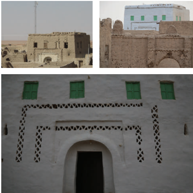
Figure 5: The Heritage Museum before and after restoration. © A. Adam
