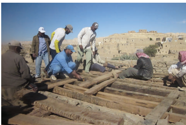
Figure 10: Fixing the palm beams on the roof. © M. Mohamed
