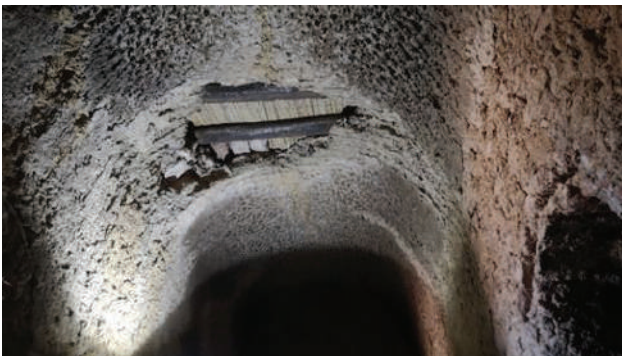
Figure 4: Room 2 - vault over the central part.
