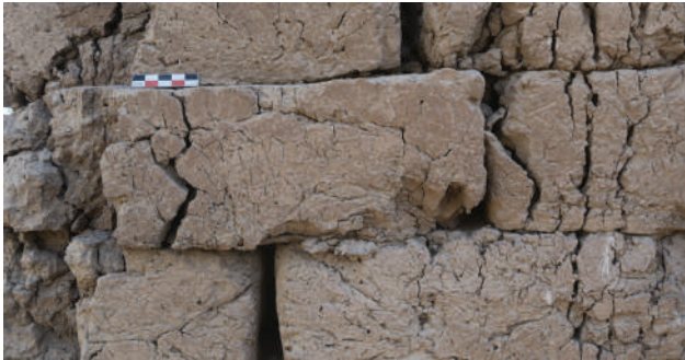
Figure 7: Detail of the masonry core: the bricks are sometimes assembled without mouna. © M. Vanpeene
