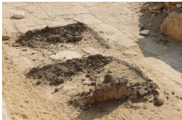
Figure 7: The small structure (see Figure 4) built right above stone slabs suffered badly in 2020.
