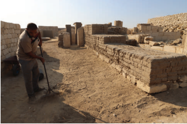
Figure 10: Levelling of the ground around the structures for proper drainage and the recovery of the stone wall basement.
