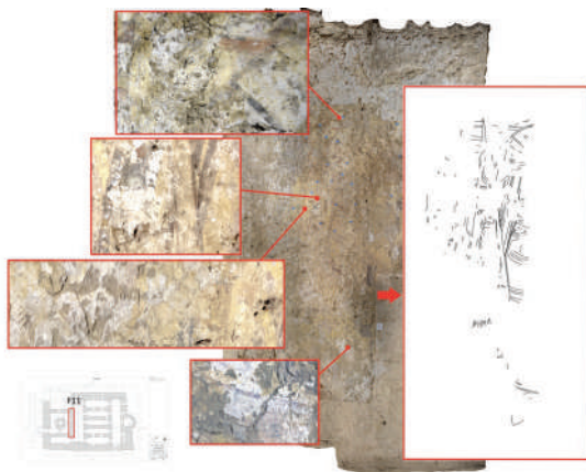
Figure 4: F11 wall. Result of the stratigraphic test. © PCMA, University of Warsaw, A. Chlebowski, M. Skarżyńska
