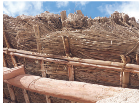
Figure 9: Traditional roof at village of Huaviña. © J. Quiroz Bravo, 2023
