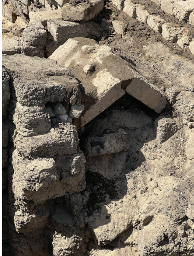
Figure 5: A feature spanning a cell that was stabilized.
