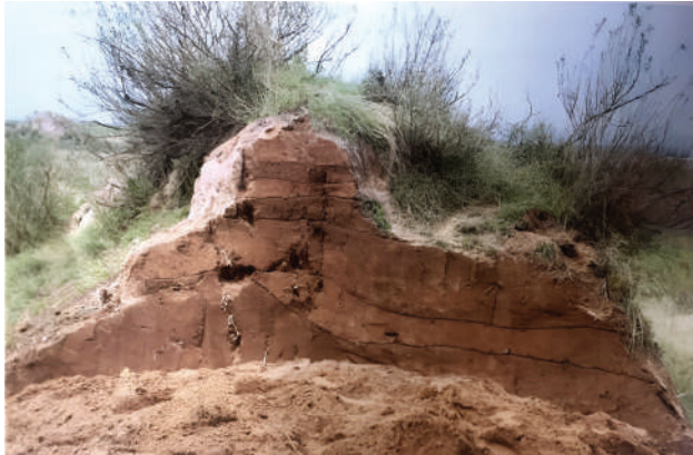
Figure 4: Stacking Earth Great Wall. © C. Xue, "Research on Construction Technology of the Great Wall in China", PhD Thesis, Northwestern University, 2018
