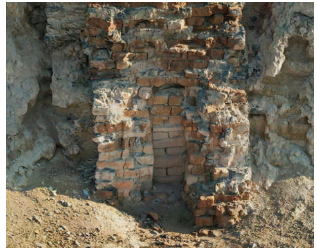
Figure 4: Water drainage in the Ezida Temple.
