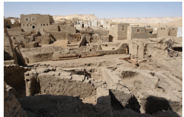
Figure 5: Severe structural degradation. © M. Mohamed
