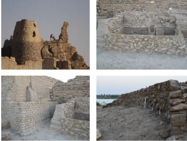
Figure 9: Walls and towers maintenance. © A. Adam
