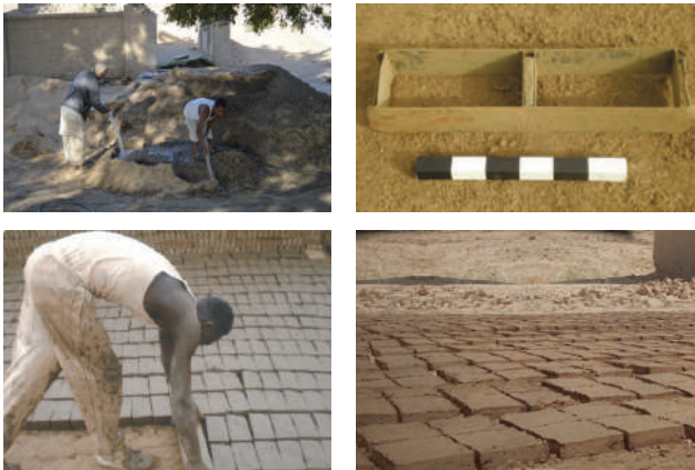
Figure 6: Preparing the mud brick for restoration. © A. Adam
