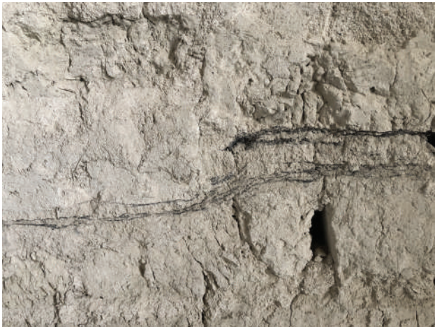
Figure 6: Layers of bitumen in earth masonry at the Nimakh Temple in Babylon. © M. Achenza
