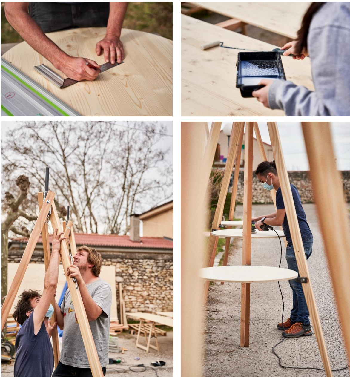
Figure 3. Photographs of the first week of construction in the retirement home, construction of totems in wooden cleats with the students Nîmes, 2021© Thomas Heydon.
