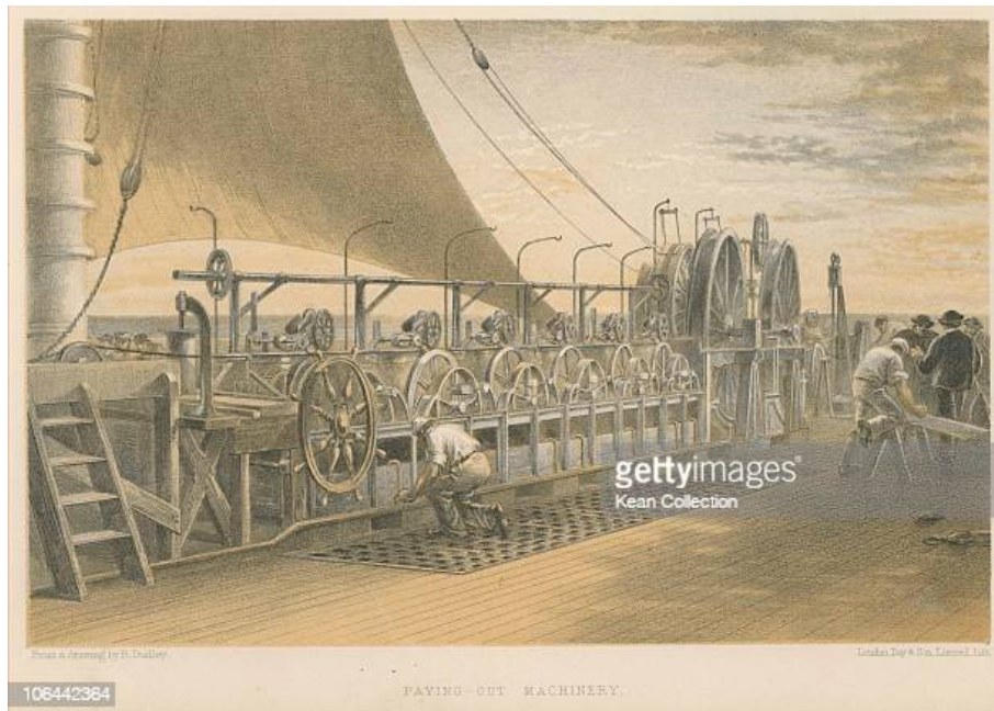
Figure 5: Paying out the transatlantic submarine telegraph cable in 1865
