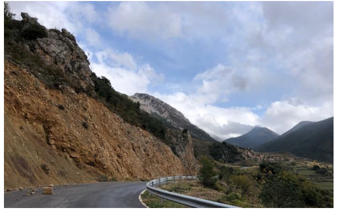
Fig 8. Landslide on a road in Alt Urgell (@RicardMoren, 2019)
