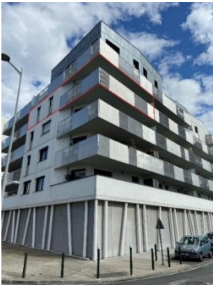
Figure 1: Photograph of the apartment, highlighted in red, from the street.
