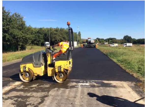
Figure 3.9: Laying (left) and compacting (right) of the VTAC 0/6 without crumb rubber.
