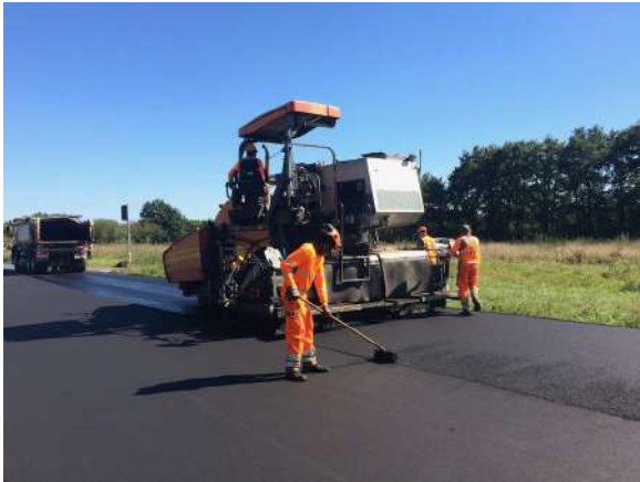
Figure 3.9: Laying (left) and compacting (right) of the VTAC 0/6 without crumb rubber.
