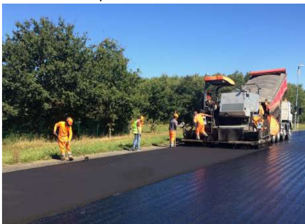
Figure 3.8: Laying (left) and compacting (right) of the VTAC 0/6 with crumb rubber.
