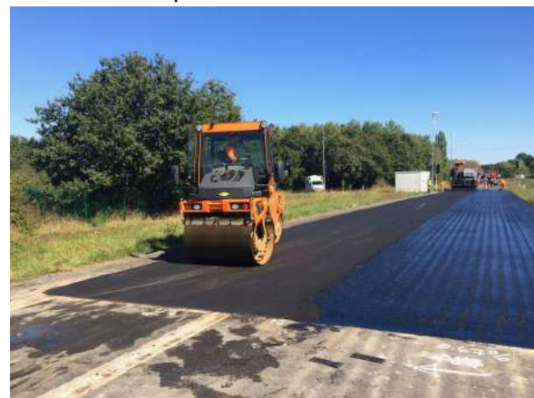
Figure 3.8: Laying (left) and compacting (right) of the VTAC 0/6 with crumb rubber.
