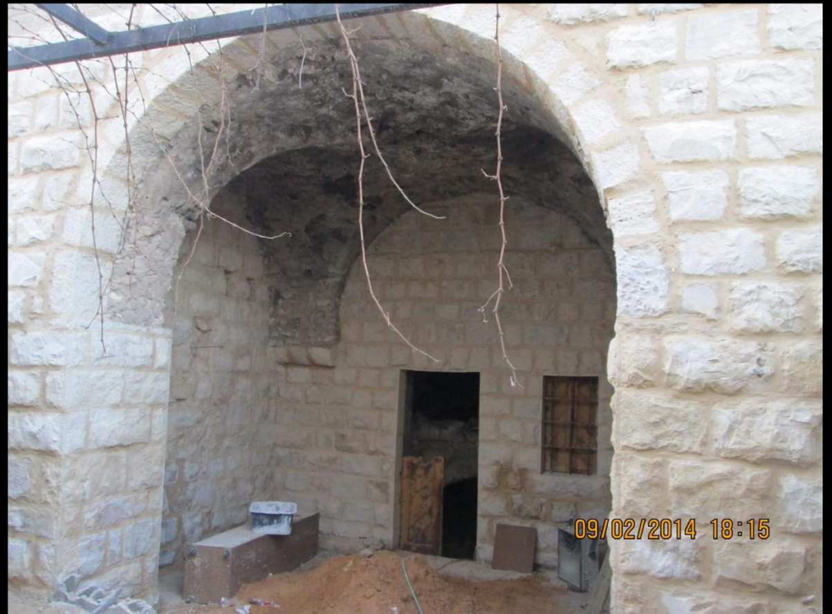
1. 1 st stage of Renovating Mazen Iwaisi's Traditional House in 2014 (courtesy Monther Iwaisi 2014).
