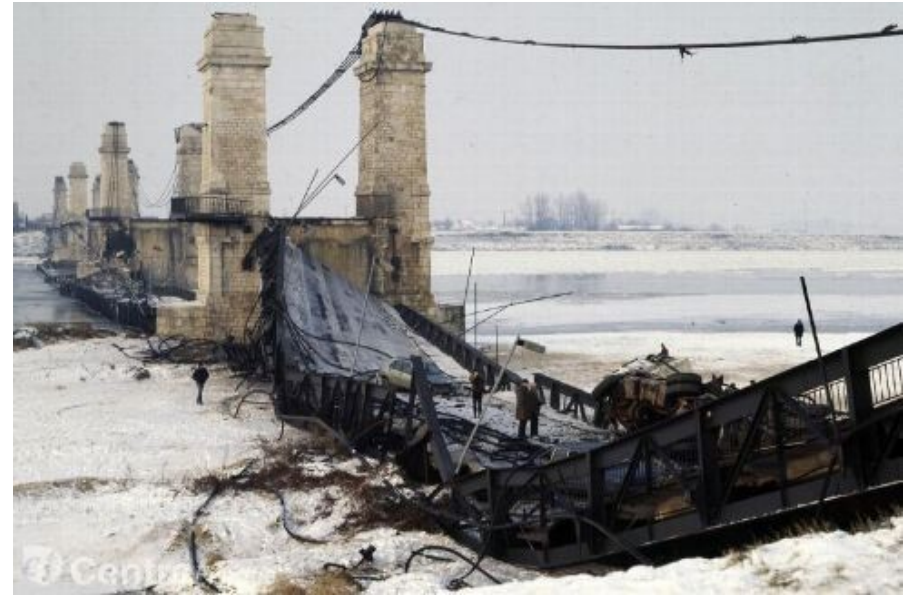
Sully Sur Loire bridge collapse on January 1985
