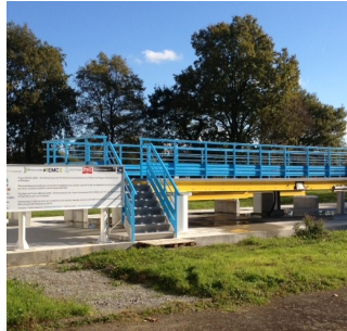
Large Smart Composite Experimental Bridge
