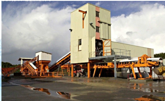
Material mixing plant
