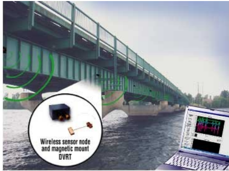
3. Wireless sensors are used to measure long-term stress and strain in civil engineering structures like buildings and bridges. (Courtesy: Microstrain Inc.)
