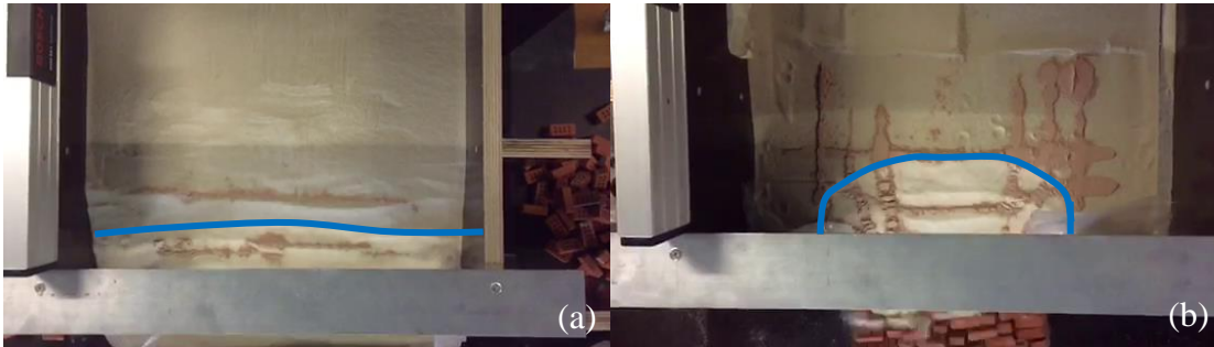
Figure 7: Top view of the failure of two walls of different lengths. (a) Straight failure line. (b) Failure curve.
