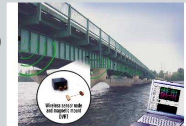
3. Wireless sensors are used to measure long-term stress and strain in civil engineering structures like buildings and bridges. (Courtesy: Microstrain Inc.)
