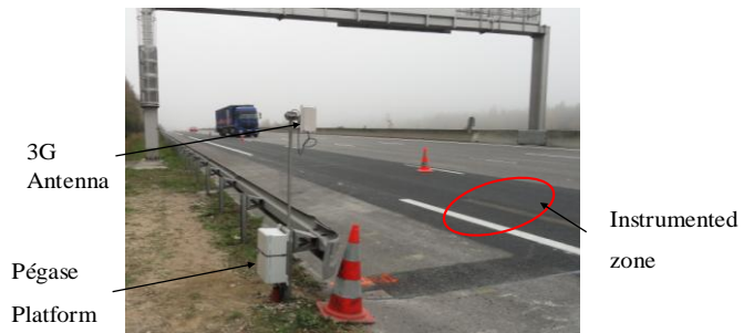
Fig. 7. View of the Instrumented Section and Data Monitoring System.
