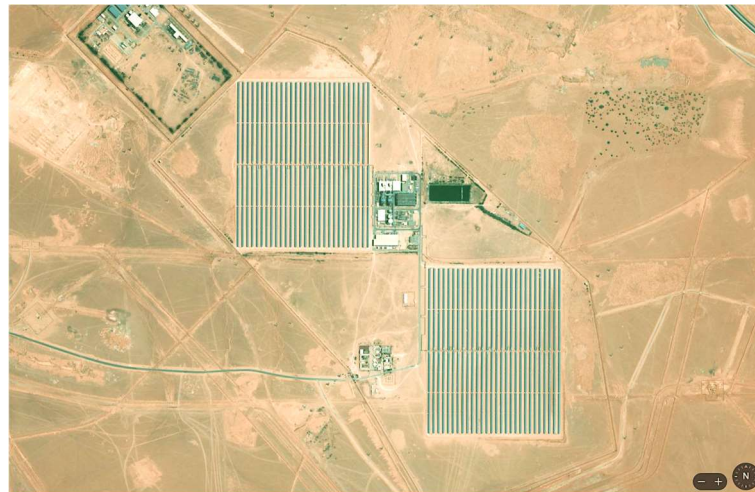
Figure 5. Satellite image of the Hassi R'Mel power plant.
