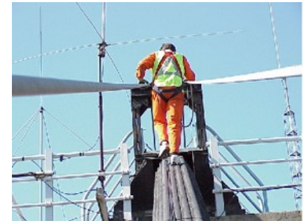
Human cable inspection
