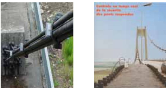
Figure 3: Iseron and Tancarville bridges
