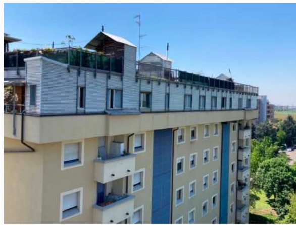
Figure 2. Public housing, Cinsello Balsamo. Source: Authors
