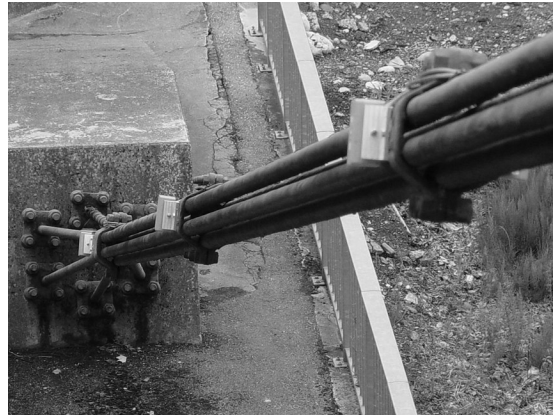
Figure 1 : initial version installed on Tancarville's bridge.
