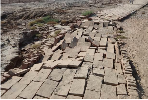
Damaged pathway between SD and L areas
