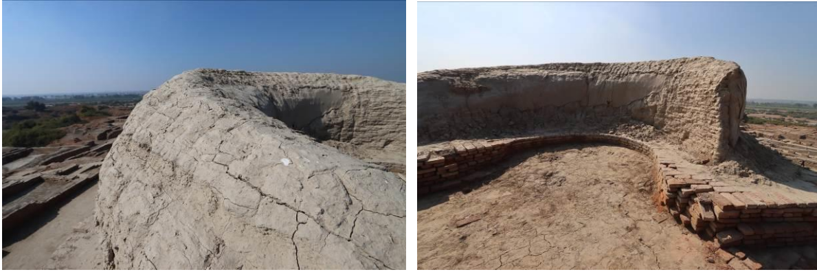
Cracks at the top and view from the inside of the stupa showing collapsed sacrificial layer.
