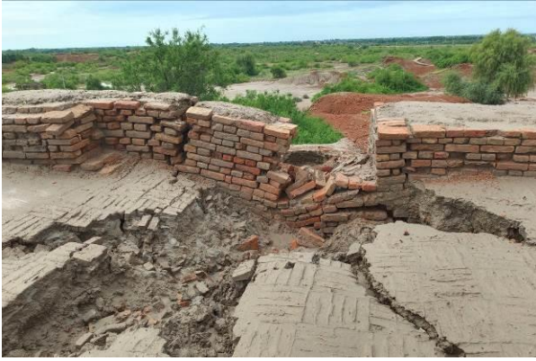
Failure of flooring-drainage at SD area © N.A.Sangha Temple at HR area, with traces of high water level
