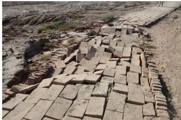
Concrete slabs of various sizes have been affected giving an idea of the violence of the runoffs
