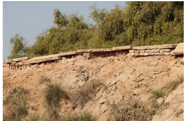
Observation of the decay of a concrete slab path and taking stock of its dangerousness, leading to the recommendation of closing this path to the public.
