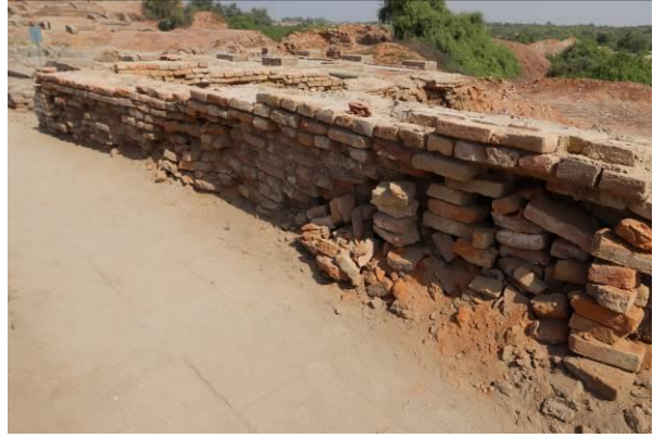
Concrete path with slope driving run-off to a wall. L area
