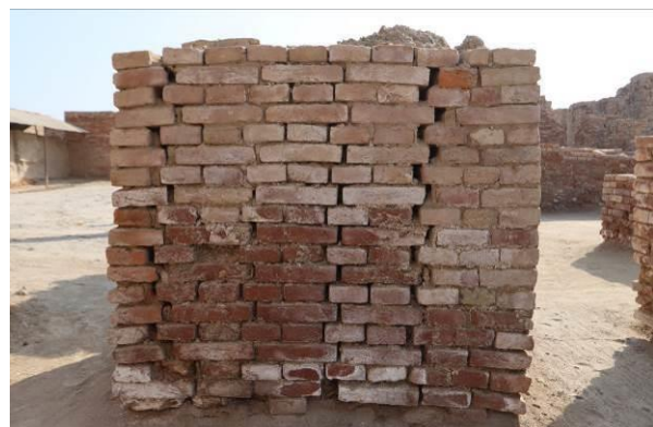
Two column types of wall (L and DKG areas) illustrating well the typical collapse process starting from the base
