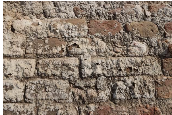
Use of mud slurry to form a salt crust against bricks
