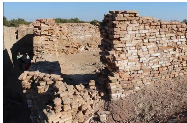
Before and after pictures of the demonstration of wall base treated temporarily with dry brick wall (without mortar)
