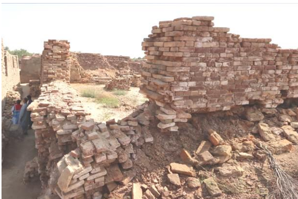
Before and after pictures of the demonstration of wall base treated temporarily with dry brick wall (without mortar)
