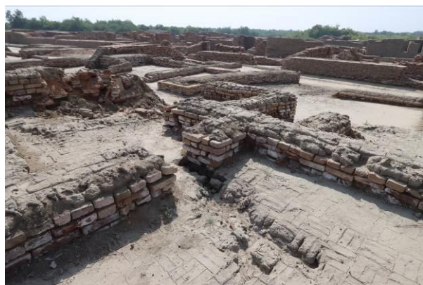
Gully type of erosion of drainage system at DK area
