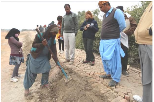
Demonstration of the rammed earth technique adapted to the construction of “high resistant shoulders” for ensuring long term durability of all types of paths (avoiding erosion at the sides), path under repair at the south east of DKG south area.
