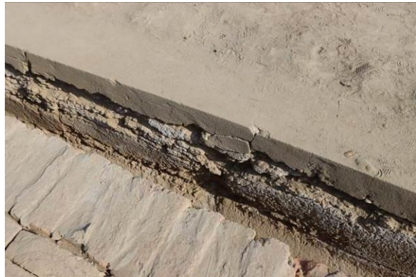
Discussion on the negative impact of a path (slope driving run-off on the wrong side) on a wall at L area
