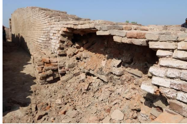
Concrete layer between the two last brick courses at HR
