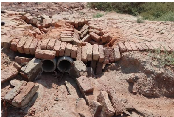
Burnt bricks paths have suffered but are easy to repair The roads at the top of the dikes have also suffered
