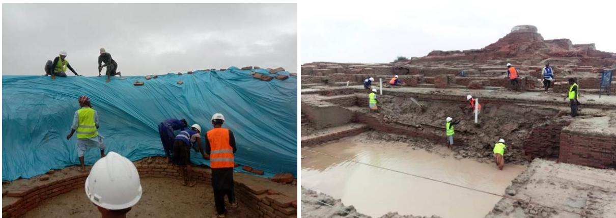
Pictures by Arch. N. A. Sangha: Left, installing tarpaulin on top of the stupa; Right, the Great bath when flooded
