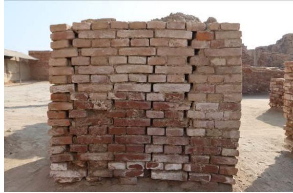
Structural cracks allowing infiltration and salt dissolution
