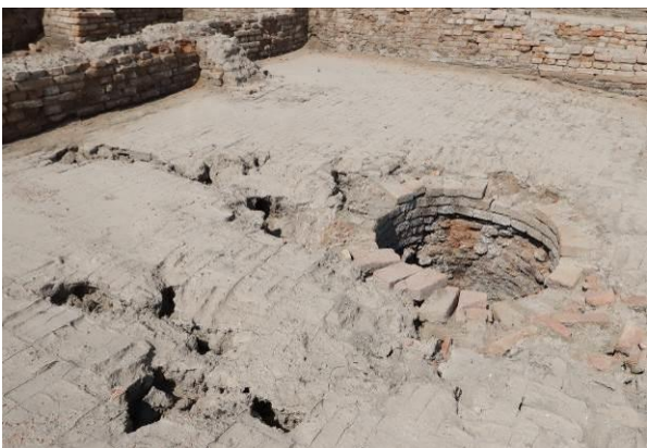
Gaps left by eroded sand under mud brick floor SV area Pushta protection affected by water infiltration HR area
