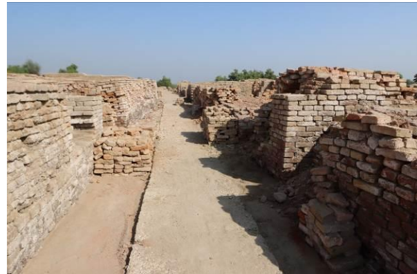
HR area, concrete slab path blocking runoff
