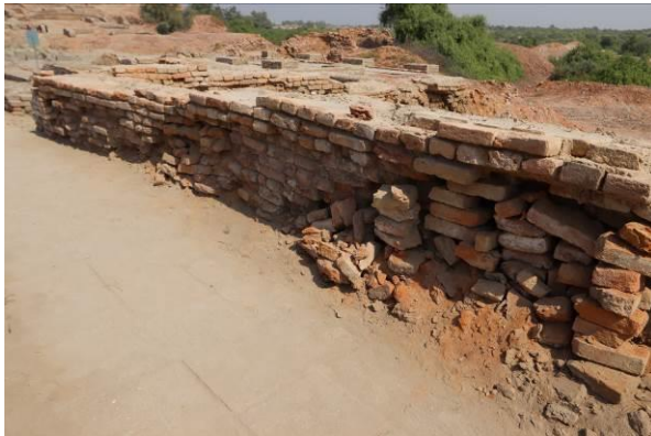
L Area, path leaning towards wall base
