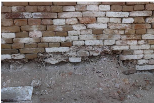
Surface crystallization and base erosion
