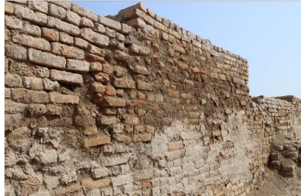
Traces of high humidity on retaining wall. SD area
