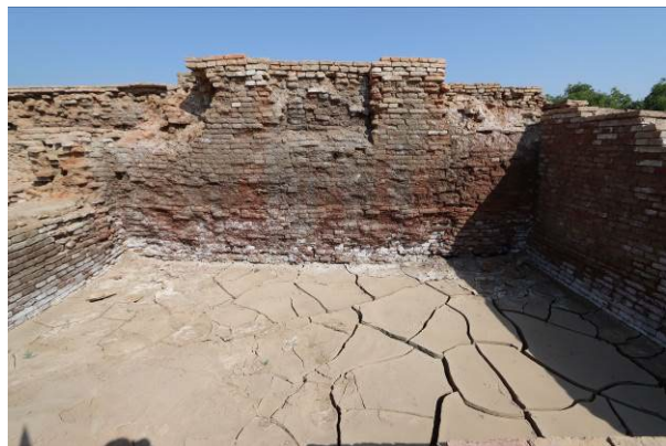
Temple at HR area, with traces of high water level
