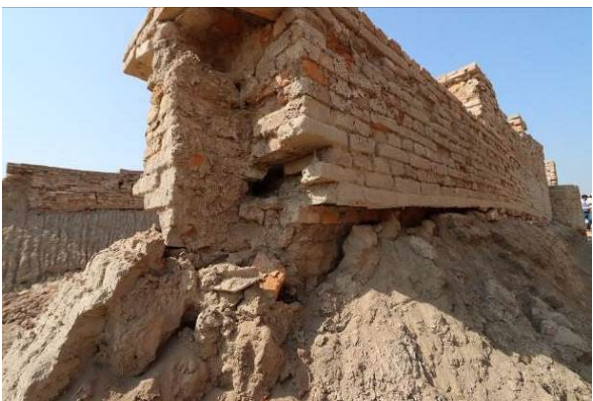
Damp proof course at DKG partly efficient
