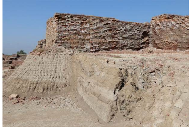
Gaps left by eroded sand under mud brick floor SV area Pushta protection affected by water infiltration HR area
