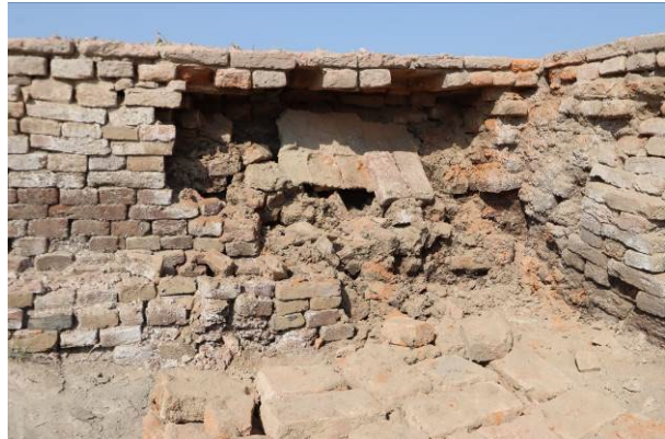
Wall collapses where salt attack has played a strong role at DKG (left) and HR (right) areas.
