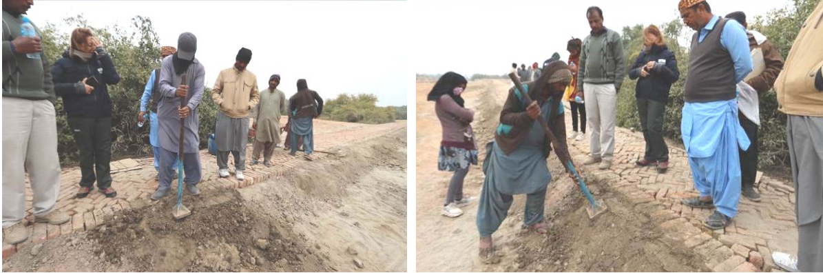
Demonstration of the rammed earth technique adapted to the construction of “high resistant shoulders” for ensuring long term durability of all types of paths (avoiding erosion at the sides), path under repair at the south east of DKG south area.
