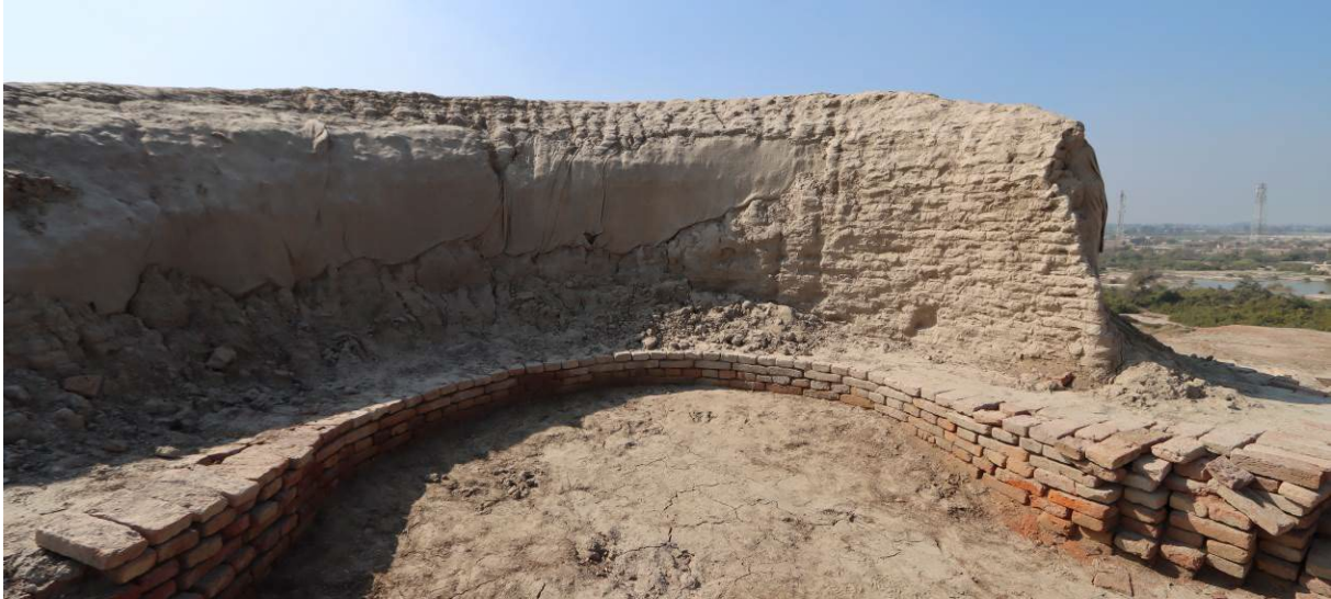
Inside the stupa, much more accessible than its outside elevation
