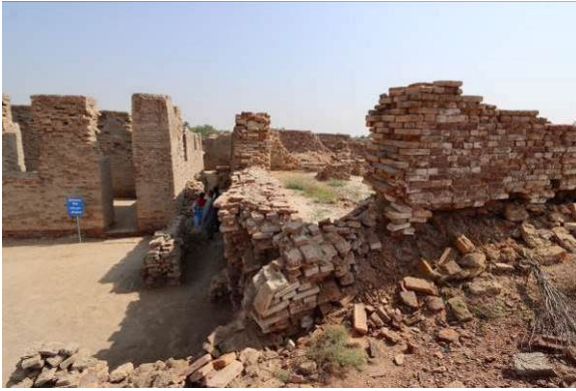
Pressure against walls by backfilling of platforms / rooms floors, DKG area (left) and SD area (right)
