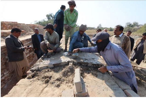
Rounded shape capping sample being prepared during field session
