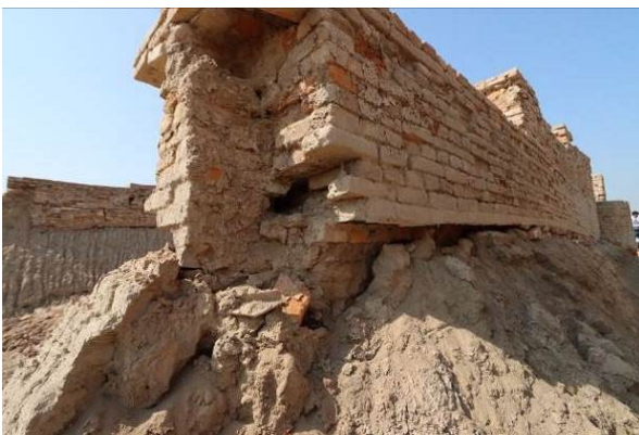
Damp proof course at DKG partly efficient
