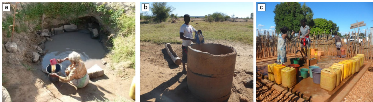
Fig. 4 Illustrations of the three types of wells sampled in the Ankazomanga basin (a) traditional well, (b) cemented well, (c) modern borehole
