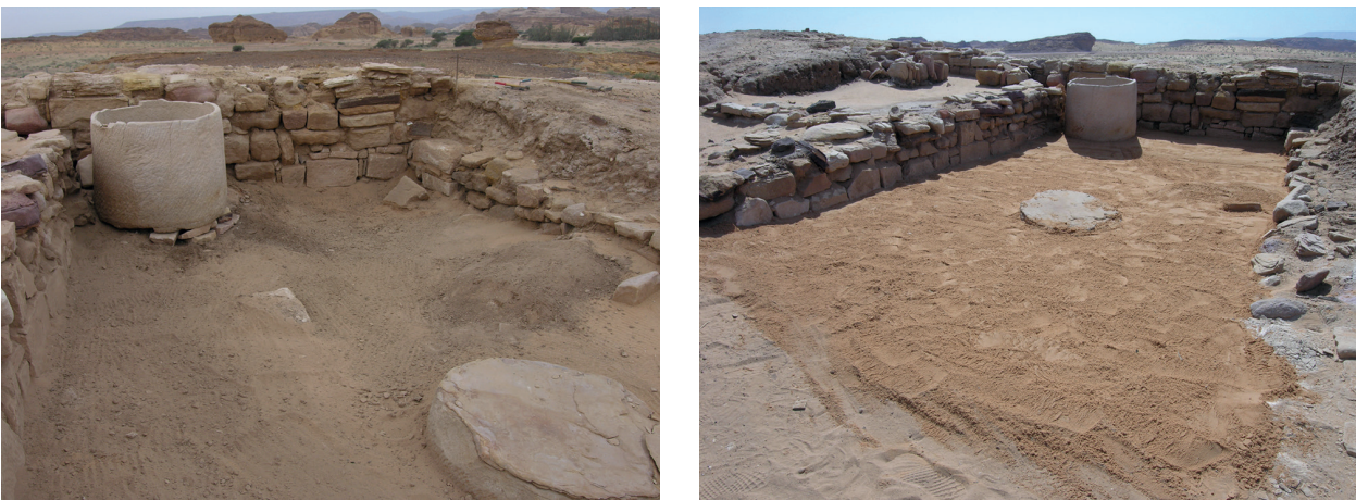
Fig. 16a–b. Wall reinforcement and backfilling in Room XI.
