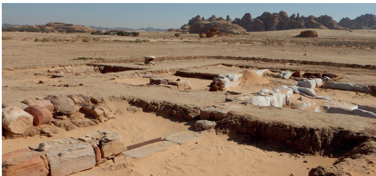
Fig. 1. Trenches A & B with backfilling both sides of threshold 91009 to compensate sand losses since last season (2022), view from south-west.
