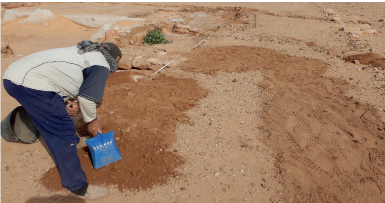
Fig. 4b. after the final backfill of the area.
