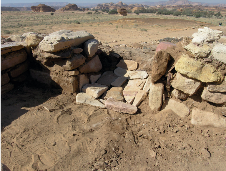
Fig. 13a. Backfilling of the doorway (Wall 34100) in Room I with small stones used to reinforce the southern doorjamb section.
