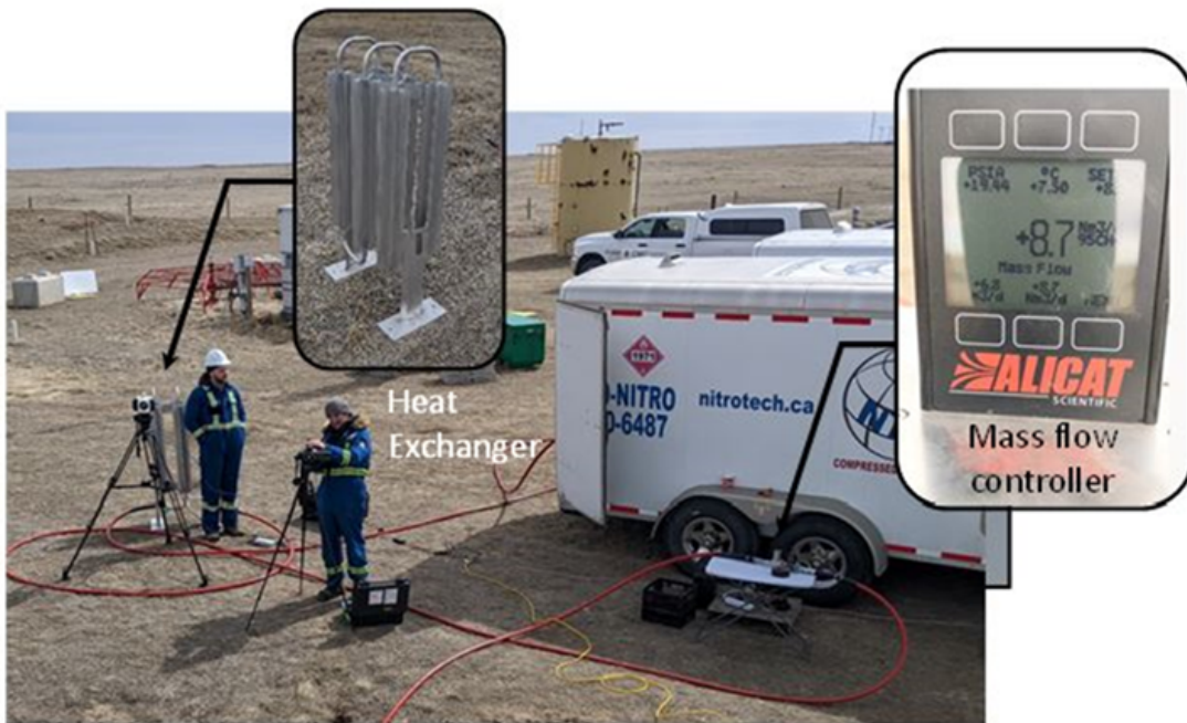
Figure 2: Controlled release set-up including heat exchanger and mass flow controller.
