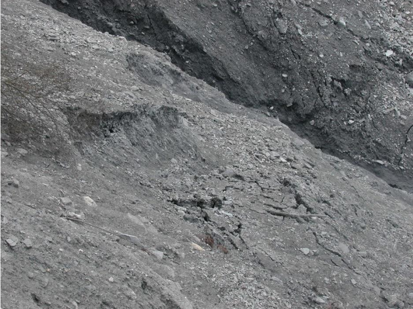
Figure 17 The ridge on the left is the top of the main scarp of an earth flow, with just below (in the middle) some blocks still recognizable, and separated by cracks
