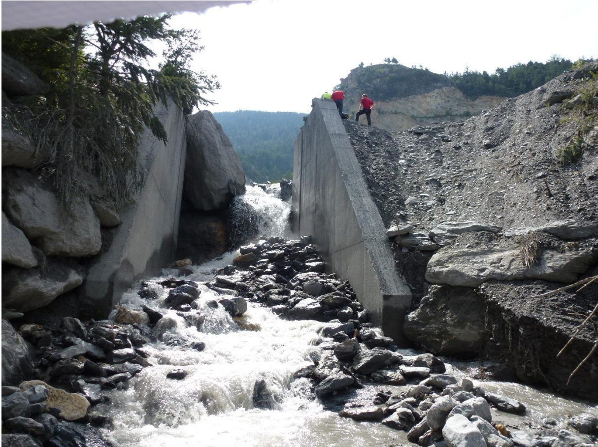
Figure 19 Slit dam closing the downstream extremity of a retention basin (Photo G. Piton)
