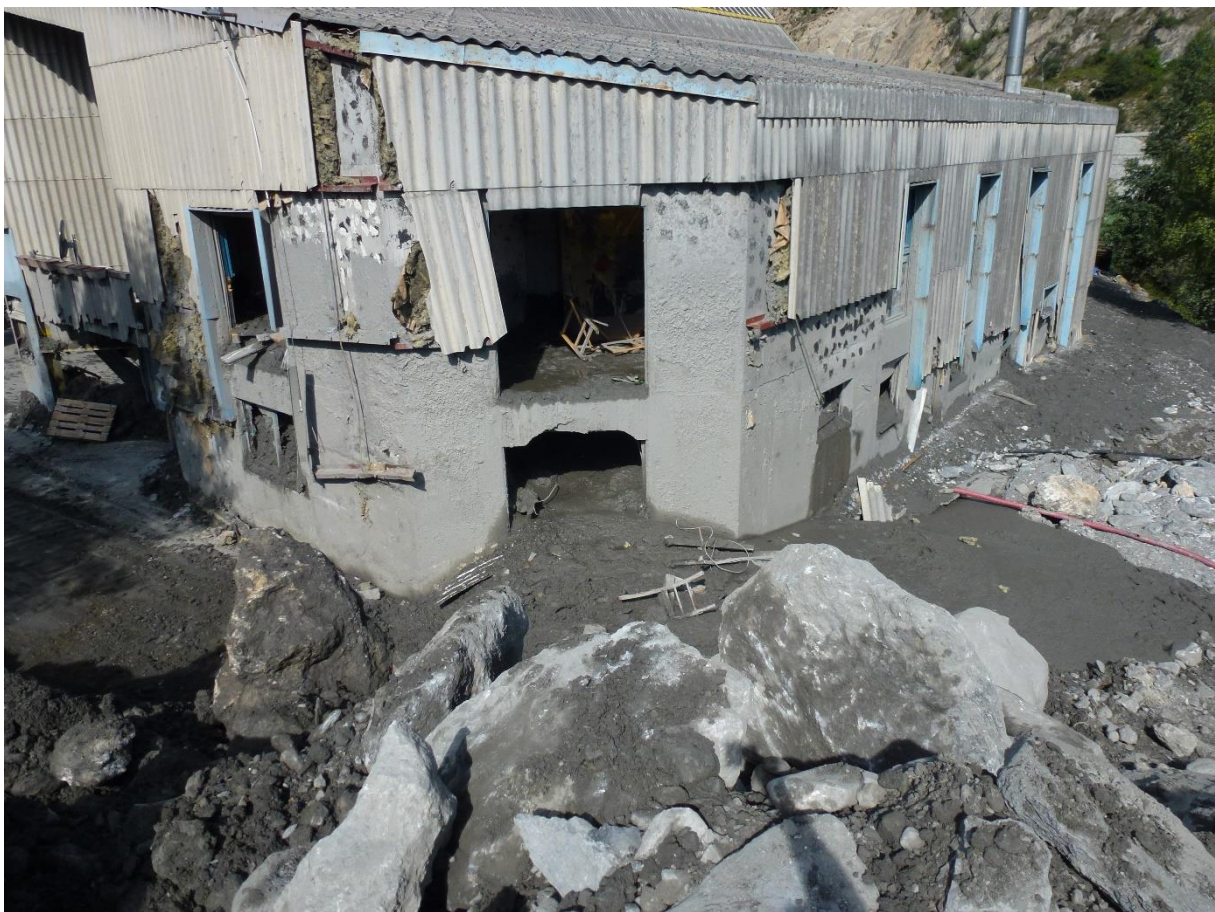
Figure 18 Example of destructive impact of debris flow that overflow its channel banks and spread on alluvial fan (photo G. Piton)
