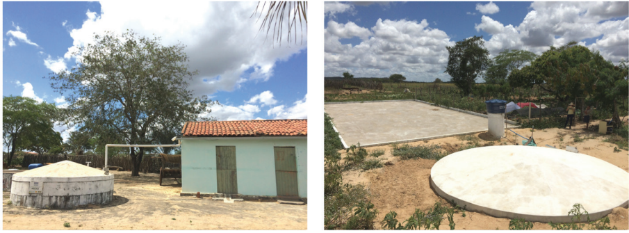
Figure 2. Main types of cisterns disseminated by the program
