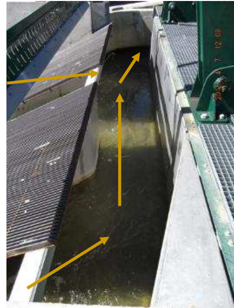
collecting bypass channel
