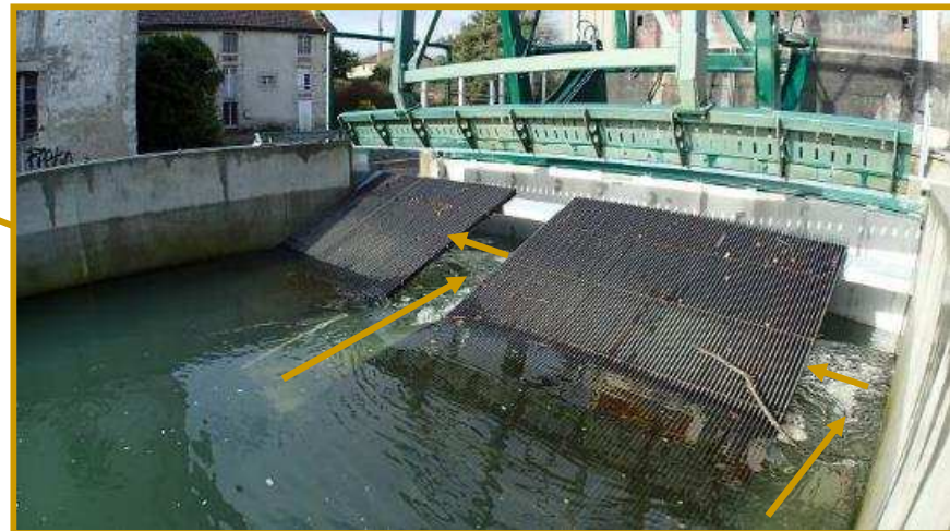
low-sloping racks with 2 bypass entrances
