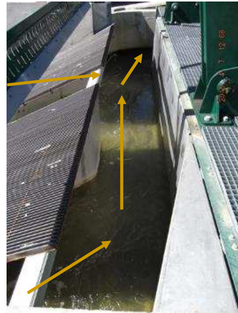
collecting bypass channel
