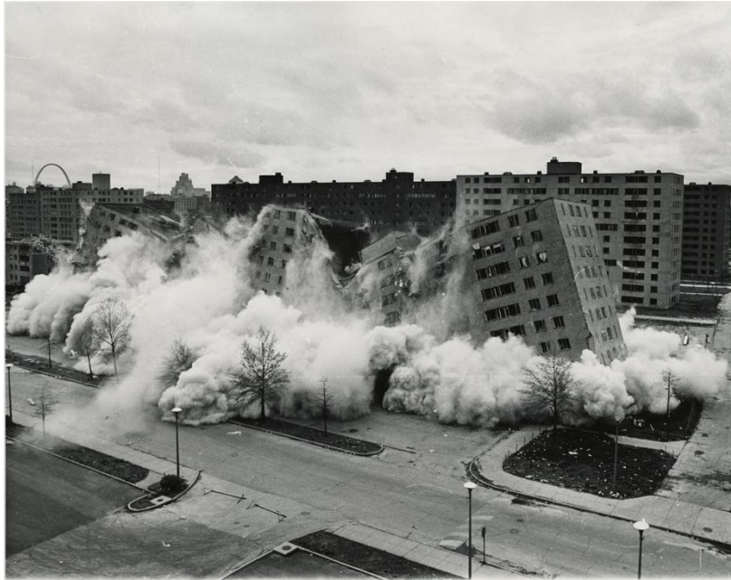
Fig.1: The second stage of demolition of the Pruitt-Igoe, April 1972. Photograph: Lee Balterman/Time & Life Pictures/Getty Image
