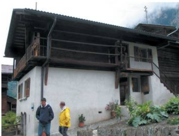
Fig. 7. The house built by Jean-Pierre Perraudin himself is now a museum in the village of Lutjero (Switzerland) (photograph by E. Rudnickaitė)
