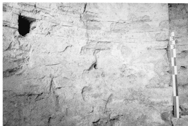
Fig. 19 : Esenköy, “site byzantin”, structure à “l’abside”, “abside”, recessed brick work .
