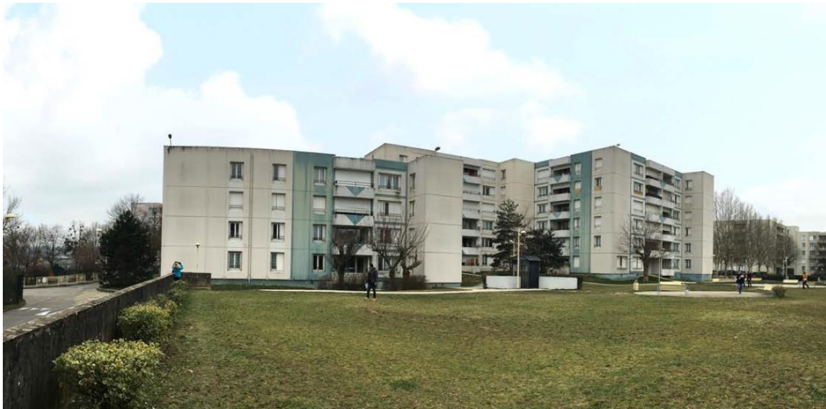
Figure 2. General view of the housing complex used to exemplify the methodology.
