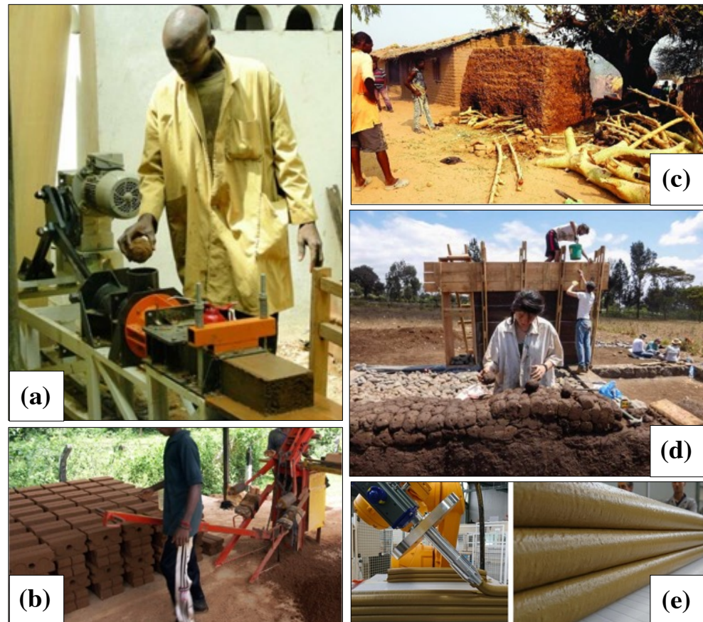
Figure 5. Example of production techniques: (a) Extrusion press prototype developed in Cameroon [11]; (b) Compressing earth with a press [12]; (c) Bricks being fired in Chembe [13]; (d) Manual technique used to build cob walls [14]; (e) Earth printing performed [15].
