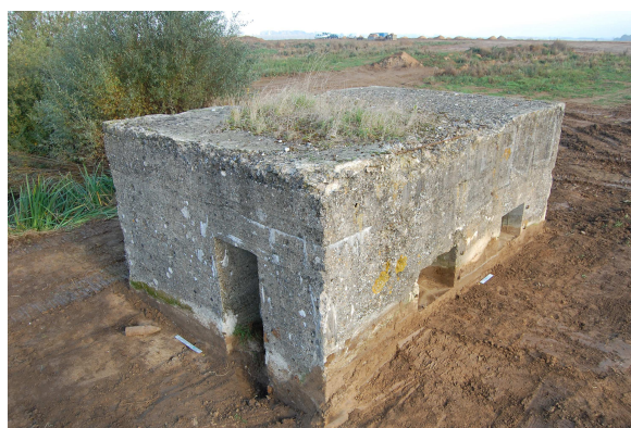
FIGURE 3 THE BRITISH PILLBOX OF AVESNES-LÈS-BAPAUME © V. MERKENBREACK, DA 62
