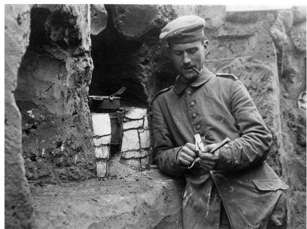
FIGURE 13 PHOTOGRAPHY OF A GERMAN FIREPLACE IN A TRENCH © PRIVATE COLLECTION A. JACQUES
