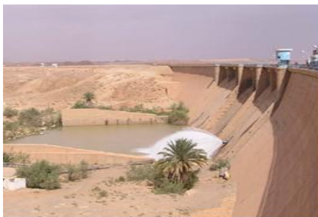
Figure 1. Overview of the dam
