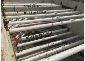
Figure 1. Les Ardoines metro station during the excavation stage – 25m of excavation
