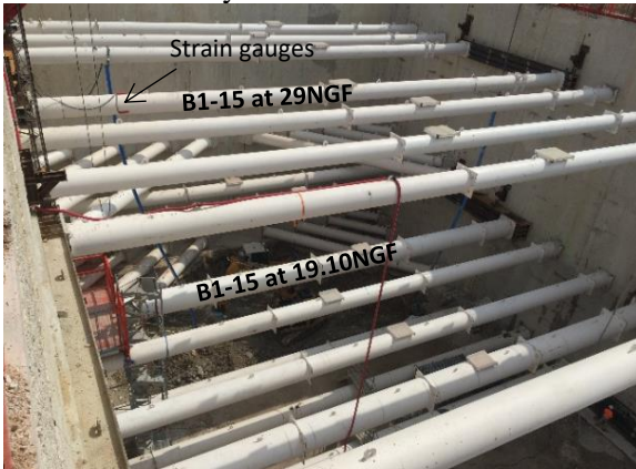
Figure 1. Les Ardoines metro station during the excavation stage – 25m of excavation
