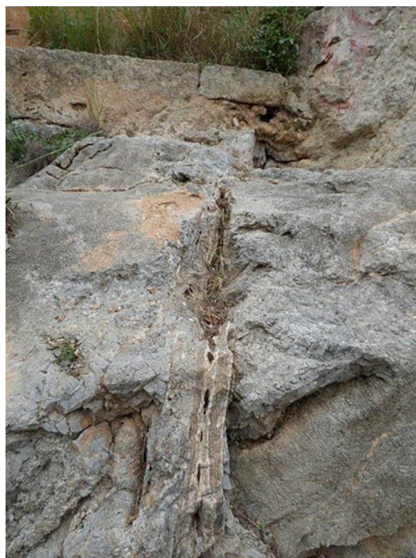
Figure 12: Solunt. General view of the calcitic lamination of the SOL 18/10 sample within substratum fracturing (photo: V. Ollivier).
