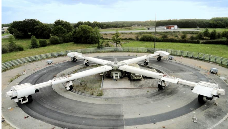
Fig. 2 The Accelerated Pavement Testing (APT) facility at IFSTTAR
