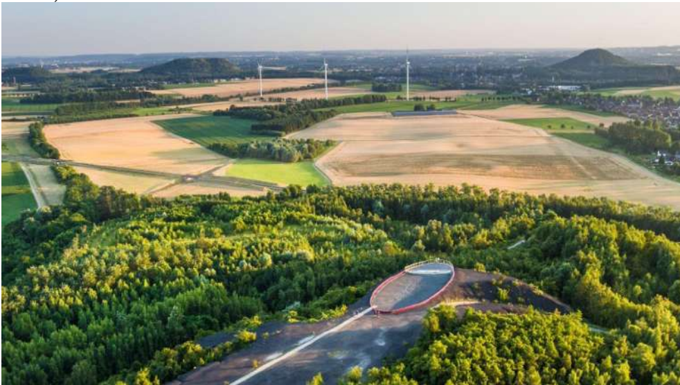
[fig.1] The Carl-Alex coal mining area in Baesweiler, Aachen (Germany) is now converted into the Carl-Alexander-Park, an attractive pole within the Grünmetropole route. © Dominik Ketz, 2020
