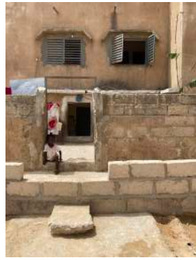
Waterproof walls in front of dwelling.
