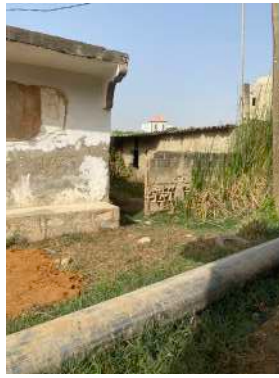
Stormwater pipe draining water from basin to canal towards sea.
