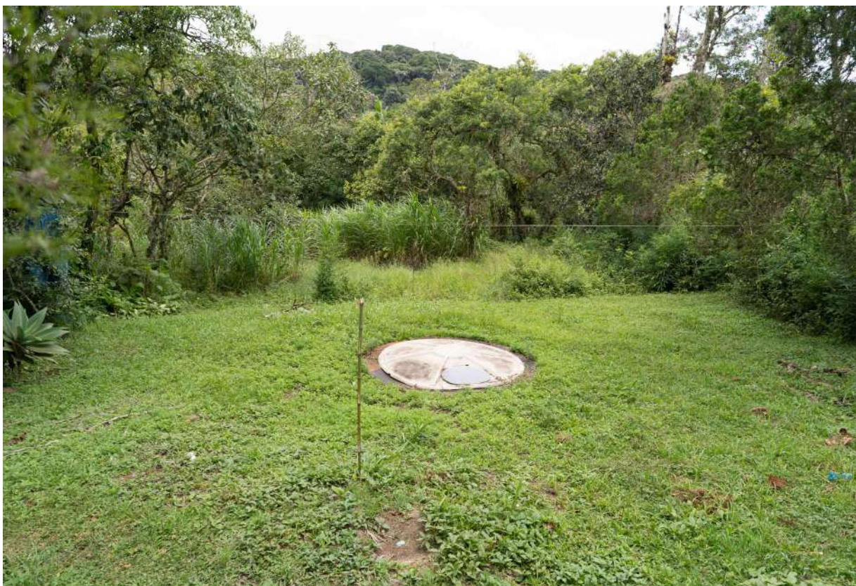
[fig.6] Sceptic pit dig by family of Comunidade KM47. Source: elaborated by the author, March 2023
