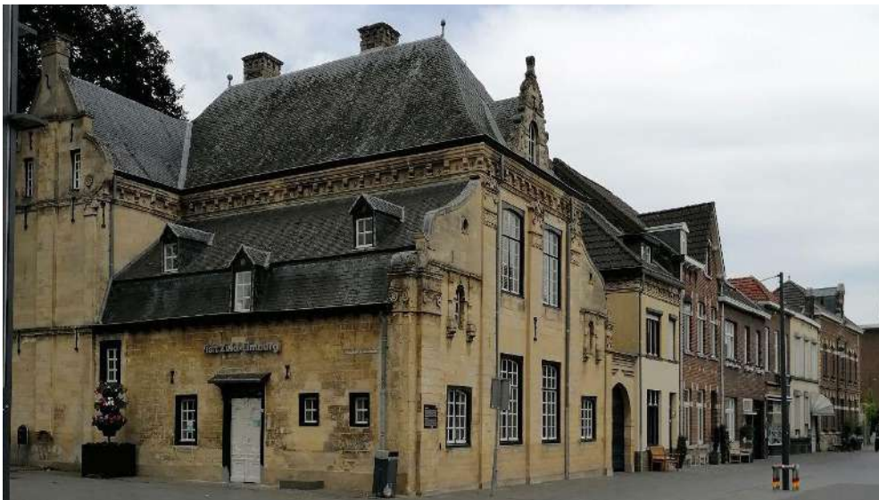
[fig.3] Characteristic building in the centre of Valkenburg in South Limburg (NL) built with local limestone extracted from an underground quarry in the region © Chiara Caravello, 2022
