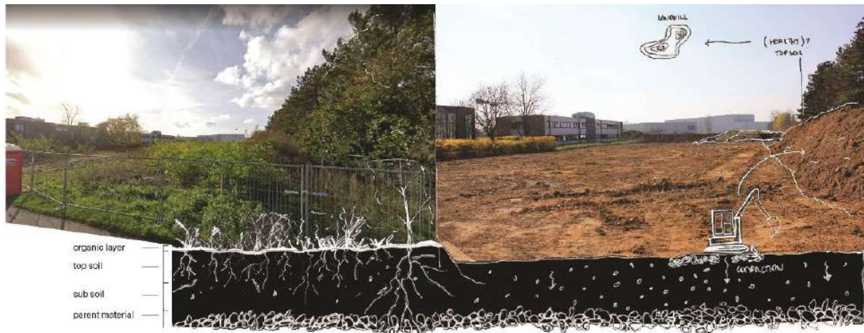
[Fig. 1] A plot at Haasrode industrial park showing a before and after excavation of valuable topsoil in preparation for the construction of a new industrial site and building. First image of Google maps, second image of March 2022 and interpretative drawing made by the author.
